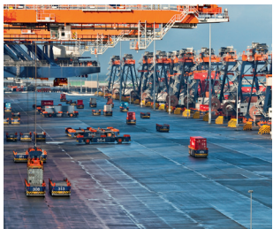
Source: Europe Container Terminals BV, Rotterdam
